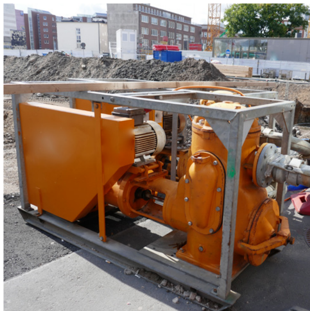
BRONBEMALING - WATER DRAINAGE
